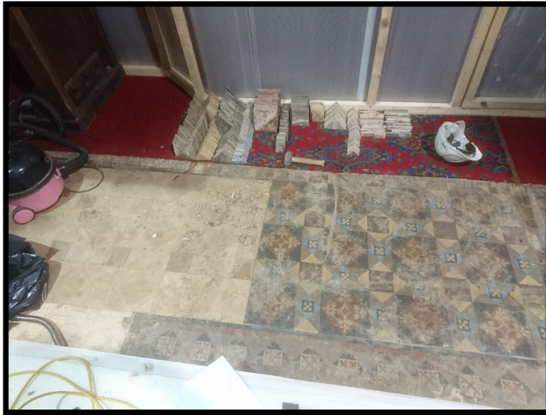
Figure 2 – Rescuing tiles underneath the carpet
