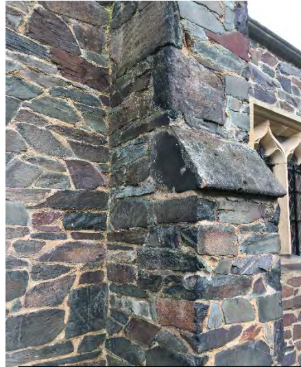
Photo 6 – Boulder stone walls
