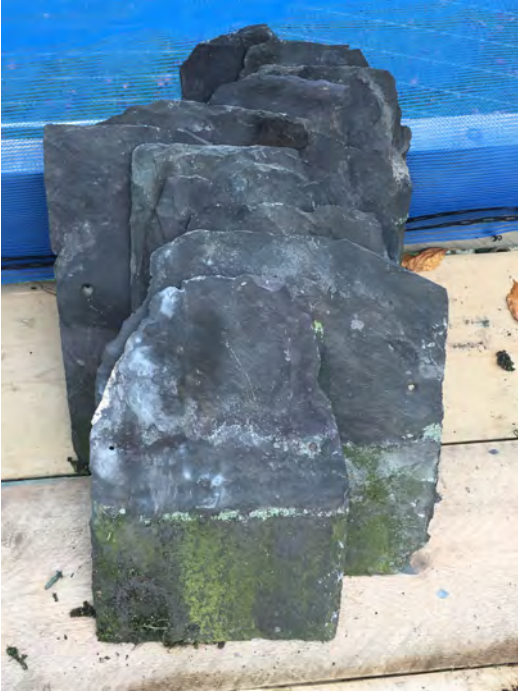
Photo 12 - Loose slates in piles before being re-fitted to St Paul's chancel
