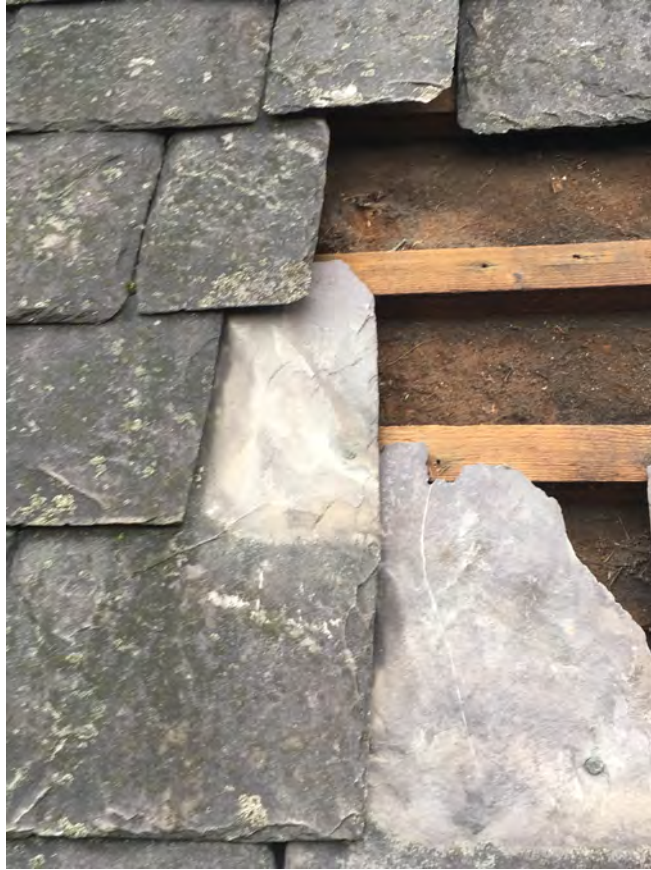
Photo 14 - Overlapping tiles on chancel roof, each one partly under the 2 above
