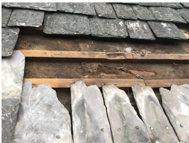
Photo 16 – St Paul's chancel roof, exposed batons and roof lining
