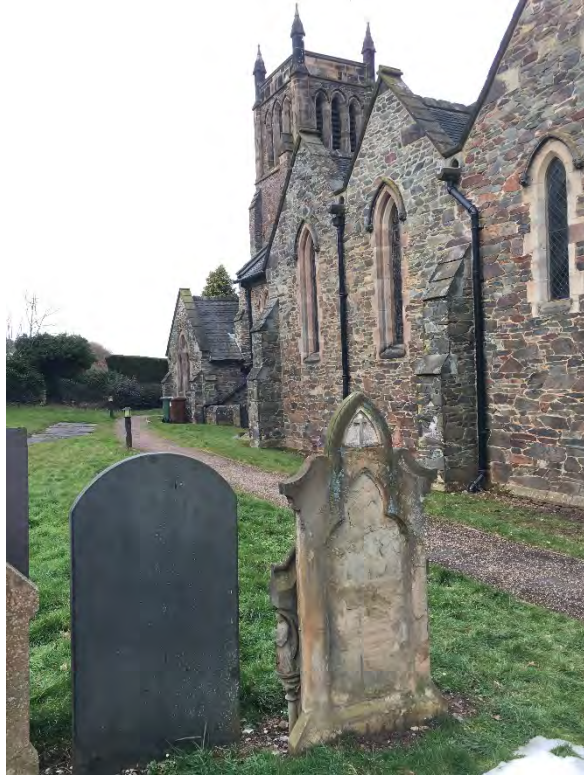
Photo 9- St Paul's gravestones, flaking softer stone on the right, Swithland slate on the left.
