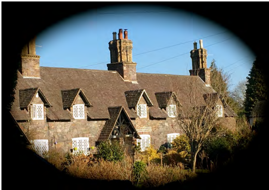
Photo 4 – Slate workers cottages, Woodhouse Eaves
