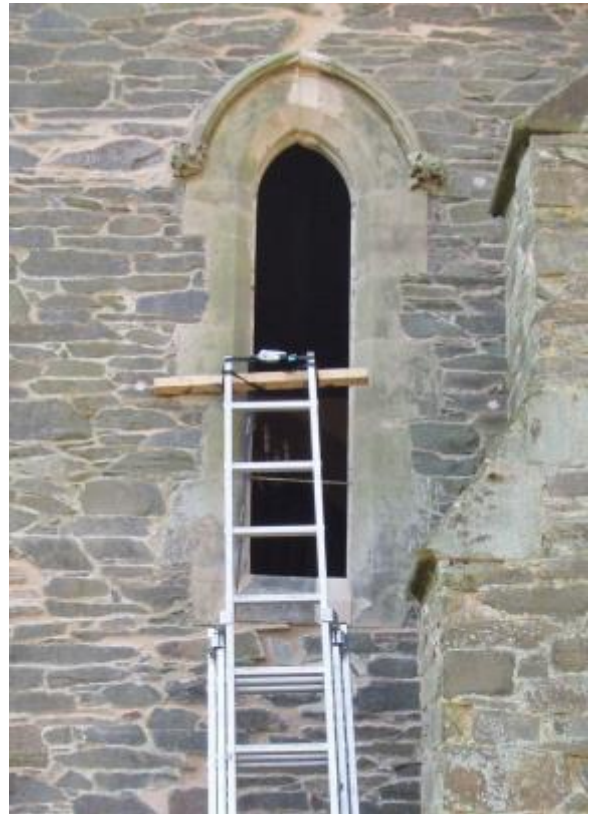
Preparing to refit the Hope window.
