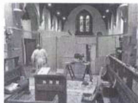
Work nearing completion in the chancel.
